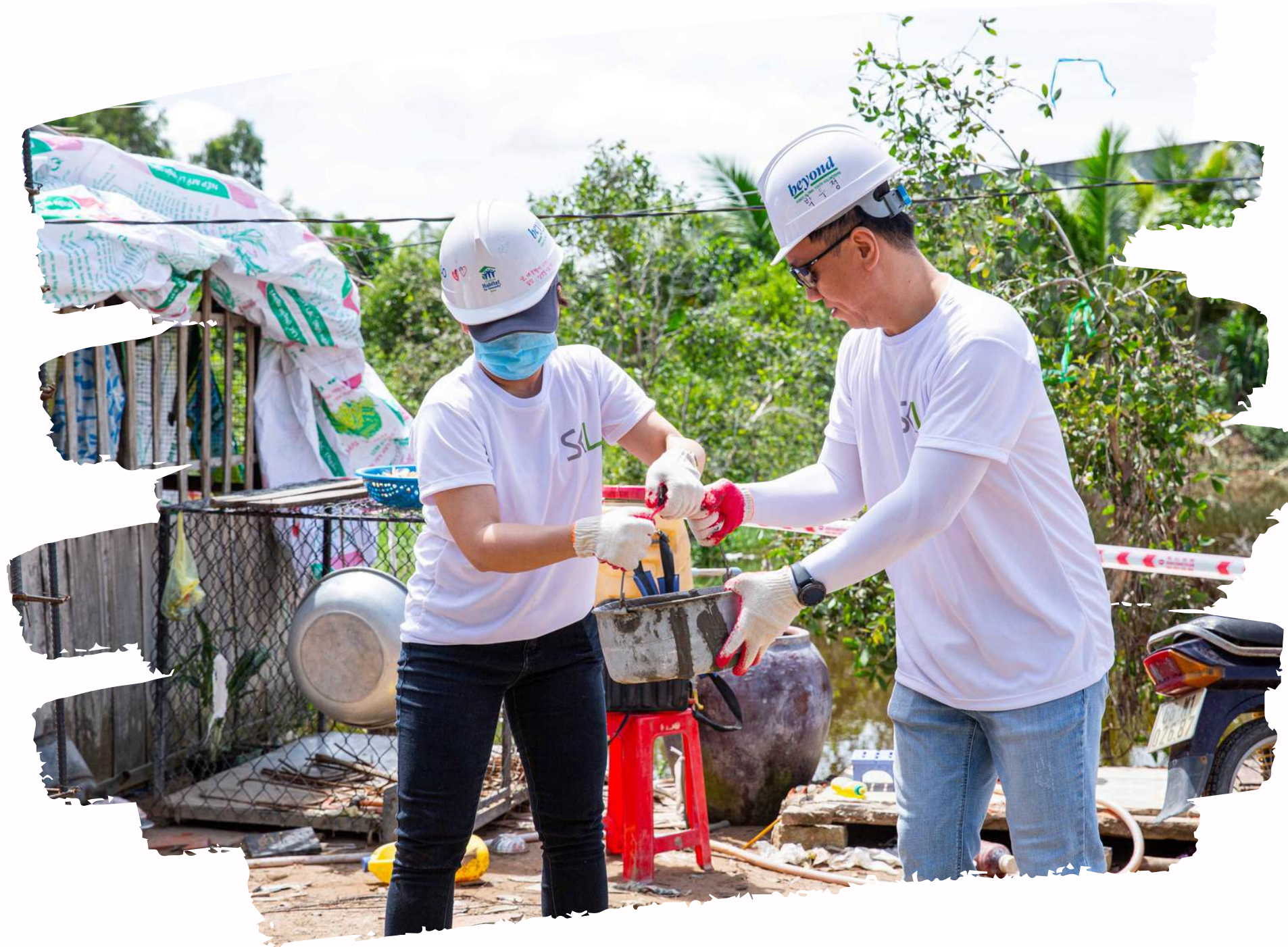
Prepare, Mix and Transport Mortar
