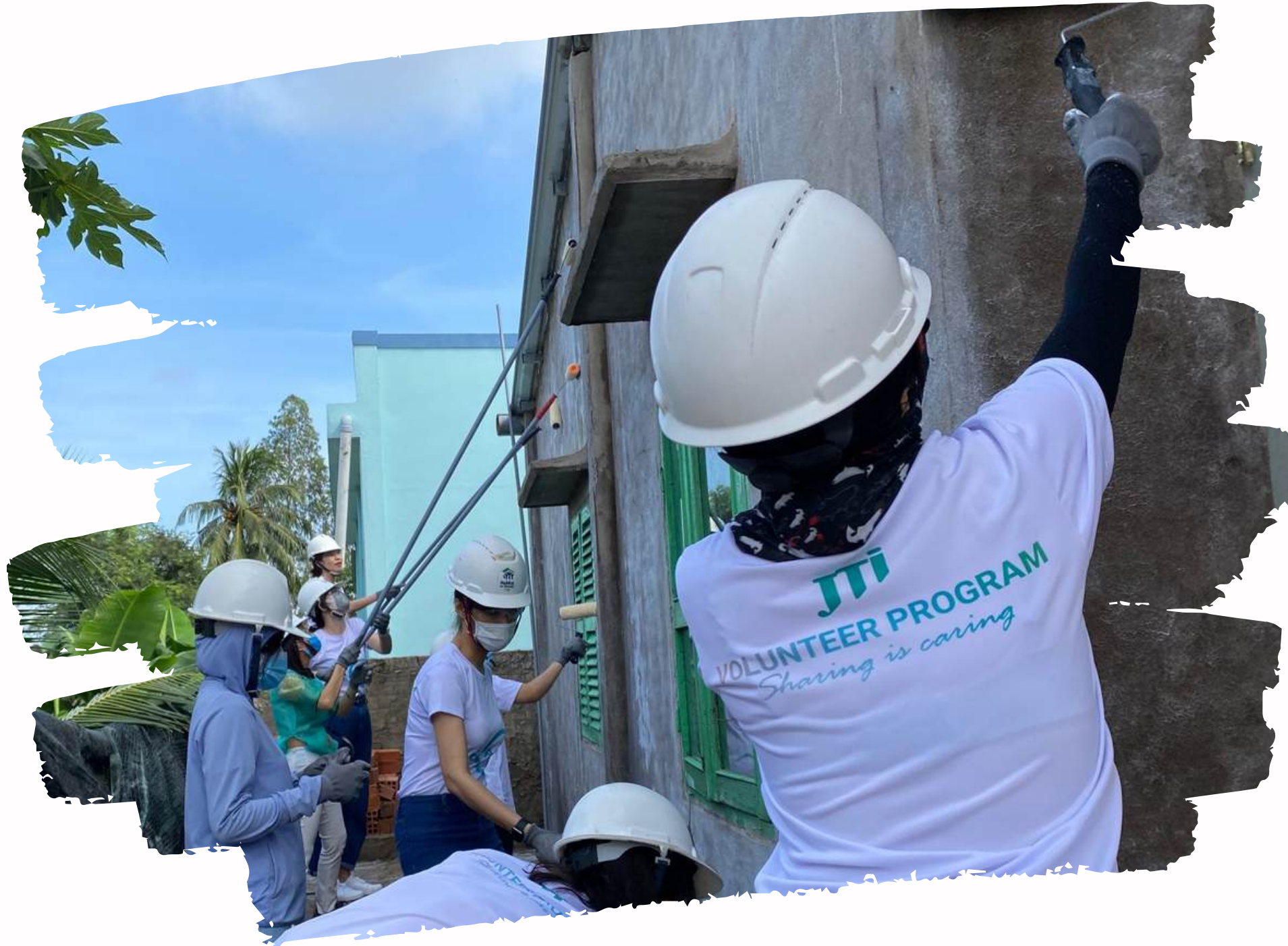
Paint the Walls
